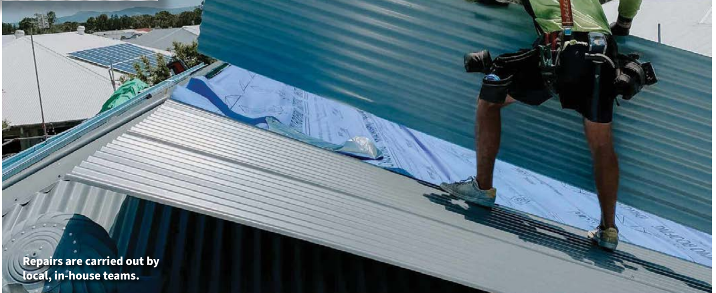
A roof inspection for hailstone dents.
