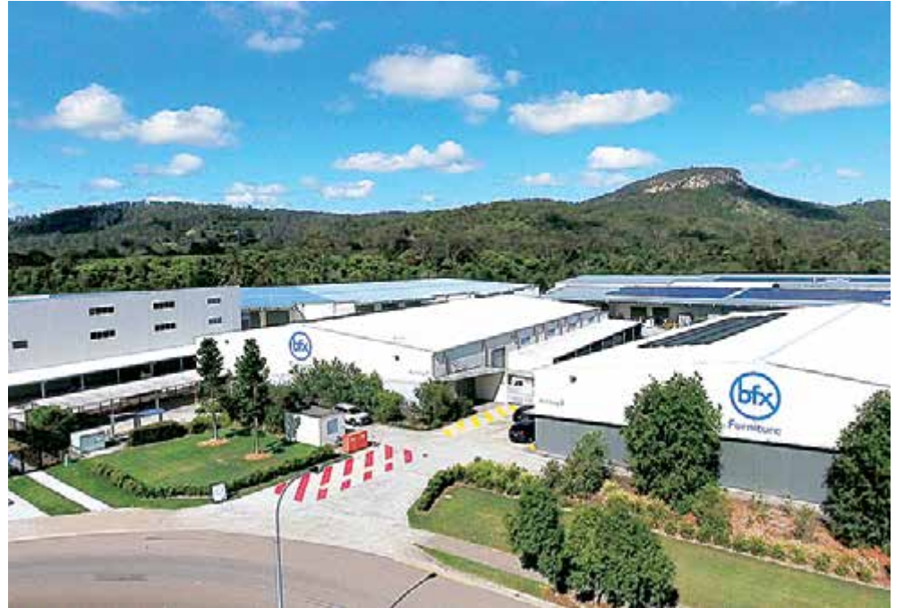
The ground-breaking $20 million expansion at Yandina Industrial Park.
