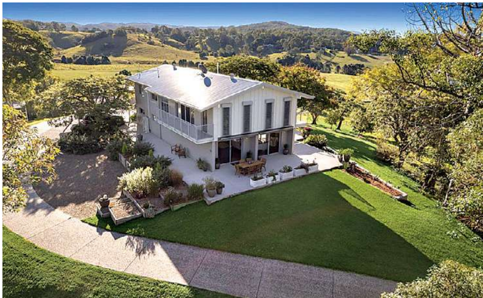
North facing, with 360 degree views, this home was stripped to its bare bones and meticulously renovated to the highest standard with a new roof, windows and doors throughout.
