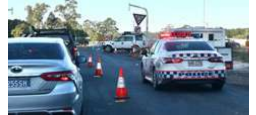
Nambour Connection Road roundabout on Sunday.
