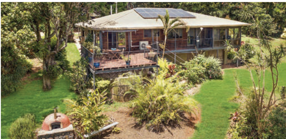
187-191 Western Avenue MONTVILLE
