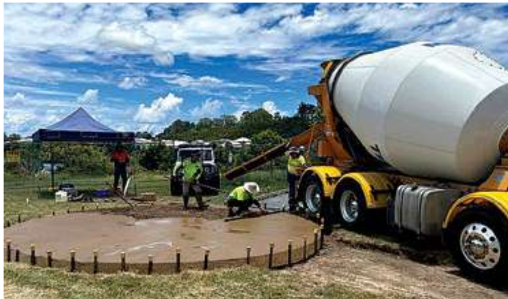
Construction in Progress at Bli Bli Cenotaph.
