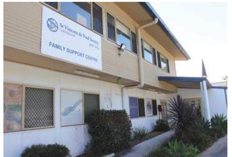
St Vincent de Paul's Family Support Centre in Rigby Street Nambour.
