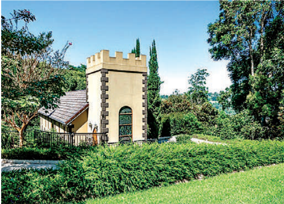
"Chapel of Angels" will be sold on or before auction on-site on June 17.
