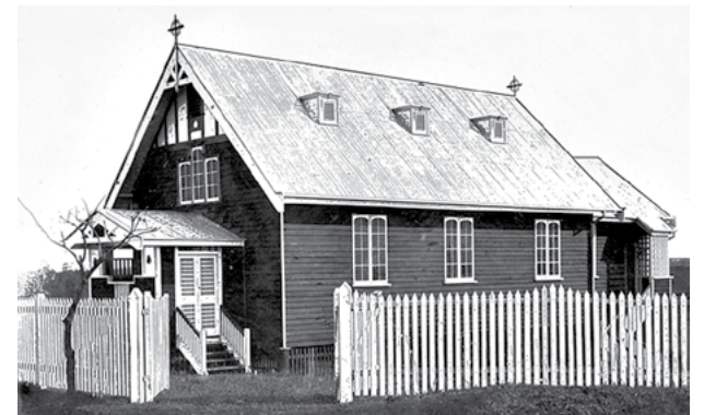
Measuring 61 feet long, including the vestry and porch, the timber and tin building cost 860 pounds to build.
