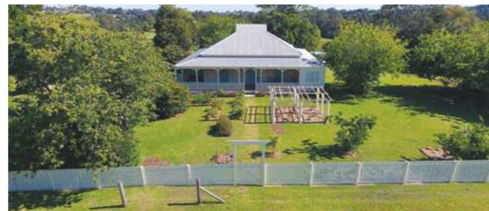
Fairview was built by the Pattemore brothers using pit sawn white beech, cut and dressed on the Maleny property. Image Courtesy Friends of Pattemore House Inc.
