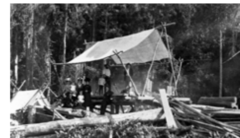
Fairview construction 1907. Courtesy Picture Sunshine Coast
