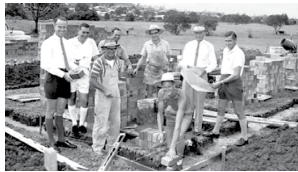
Setting the first brick, 18 February 1963. From left: Ian Hayne (Apex), Dr Allan Raine (President of Nambour Apex Club), E. 'Tibby' Scells (bricklaying contractor), Bill Blandford and Keith McKinnon (building contractors), Gavin Scells (laying brick), J.D. Grimes (Sundale Administrator 1963-1973) and Noel Parry (design and building consultant).
