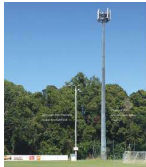
The image puts into perspective the scale of the 40 metre tower when placed alongside a 22m light pole and tree line on the Woombye Snakes Football Field. This image is a representation of the scale of the proposed tower. Note: proposed tower is to be located on the western end of Campbell St & not on the football fields.
